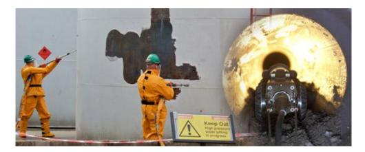
When a Midwestern crew arrives at a job site, you can be assured they will arrive with a complete inventory of specialized tank cleaning equipment. Our equipment trailers have been modified and improved through over 30 years of experience. All equipment is either air or hydraulically powered to allow working in potentially explosive environments. We provide pumping equipment that is designed to handle viscous tank bottoms. Each equipment trailer is equipped with: The Right Equipment for the Job.
